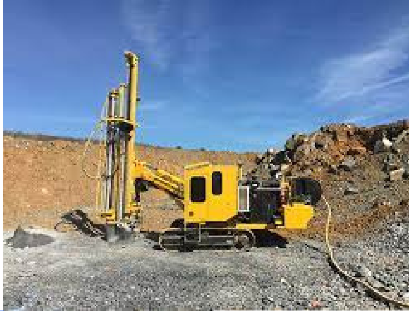
Blast Hole Drilling
