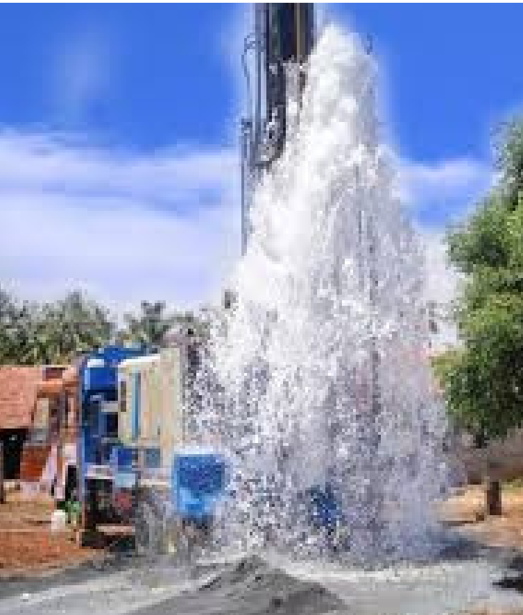
BoreHole Drilling
